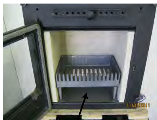
Securing screw located under grate
